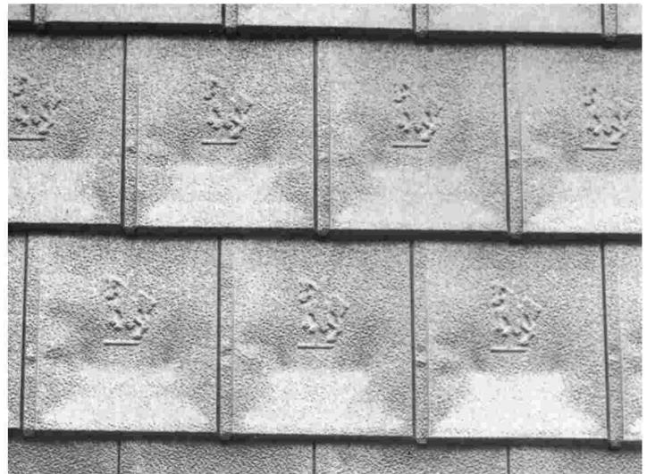
Close-up of the copper shingles used in the carousel's fascia reveals an embossed design mirroring the copper horse atop its copper-shingled roof.
