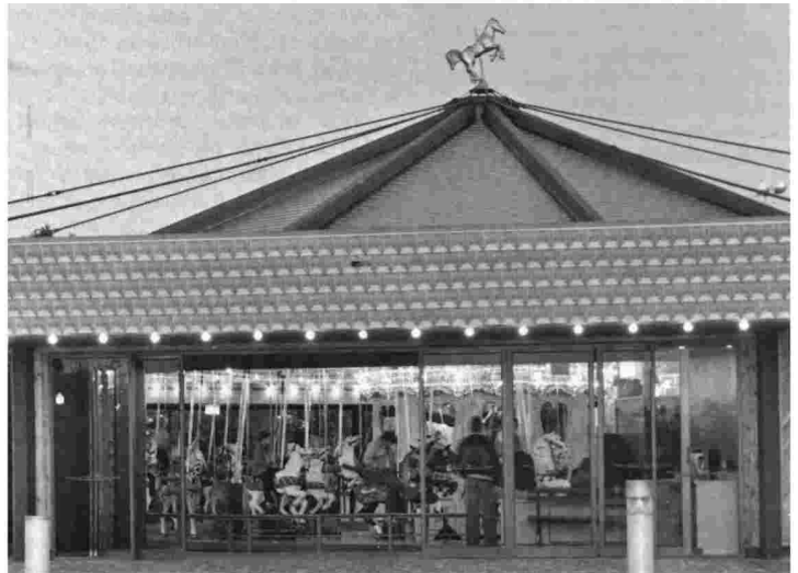
Spokane's newest landmark is a copper-topped carousel in the city's downtown Riverfront Park. The antique merry go-round is housed in a glass-walled building with a four-foot high copper fascia, a copper-shingled roof, and a copper horse. More than 10,000 copper shingles make up the glistening roof.
