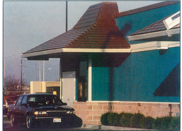
McDonald's in Kent, Washington, showing the roof made of solid copper shingles.
